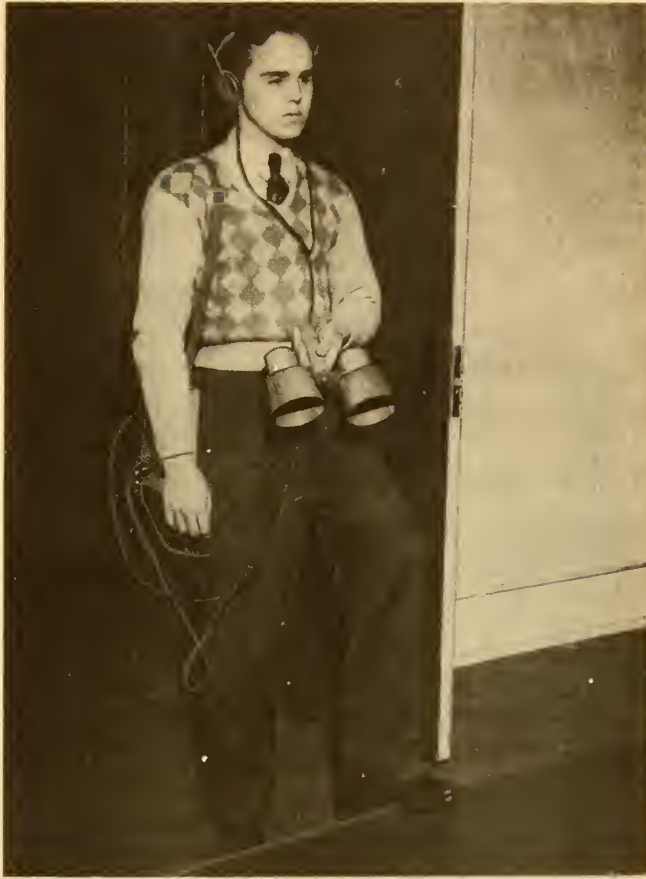
FIG. 2.6 SUBJECT CARRYING STROMBERG-CARLSON SUPERSONIC DEVICE, YA-3ST.
